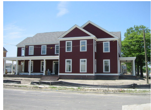
Figure 1: Image of a multi-family apartment building designed to resemble a large single-family home.
